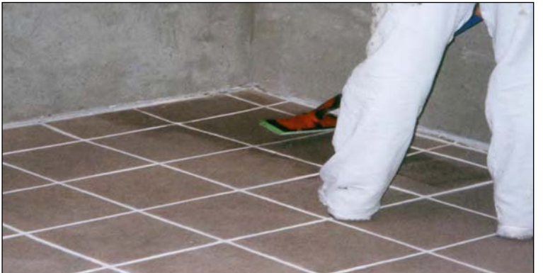
Tyfo® Sealer being applied
