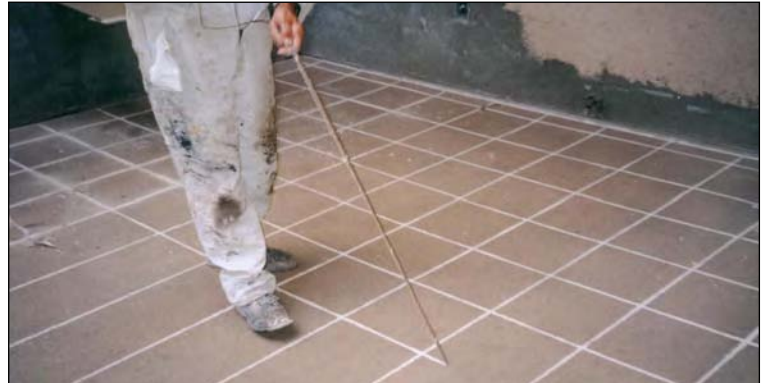
Tape, to simulate grout lines, being removed
