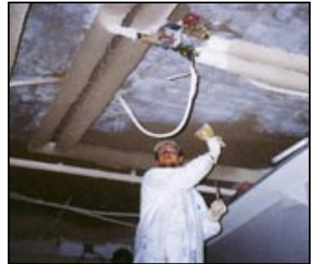
Tyfo® EI being applied around obstacles
