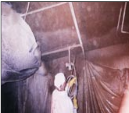
Subsequent lifts of Tyfo® VG applied
