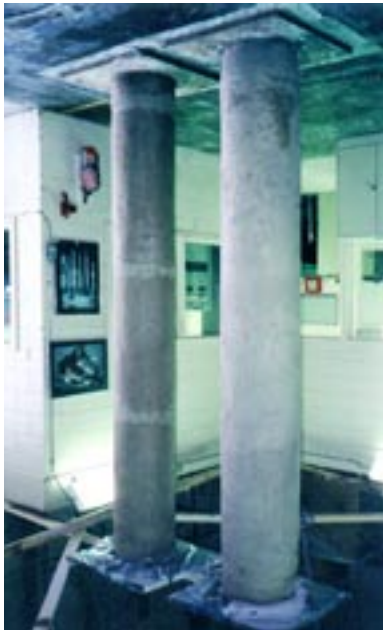
Columns to be tested
