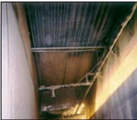
First lift of Tyfo® VG sprayed-applied
