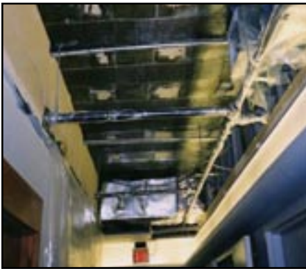
Tyfo® Carbon Composite applied
